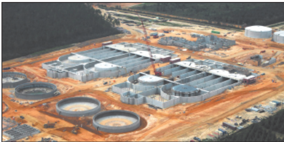
Construction site of the Central Water Reclamation Facility, showing (from top right) reclaimed water EQ tanks, the administration building, BNR basins, clarifiers, and filter structures.
