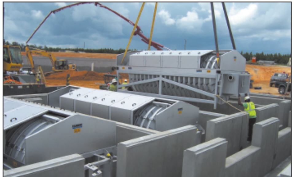
Filter installation at the Central Water Reclamation Facility in July.
