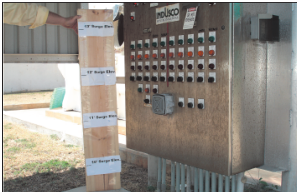
The electrical control panel at Main Street Plant, showing the storm-surge flooding level resulting from Hurricane Ivan.
