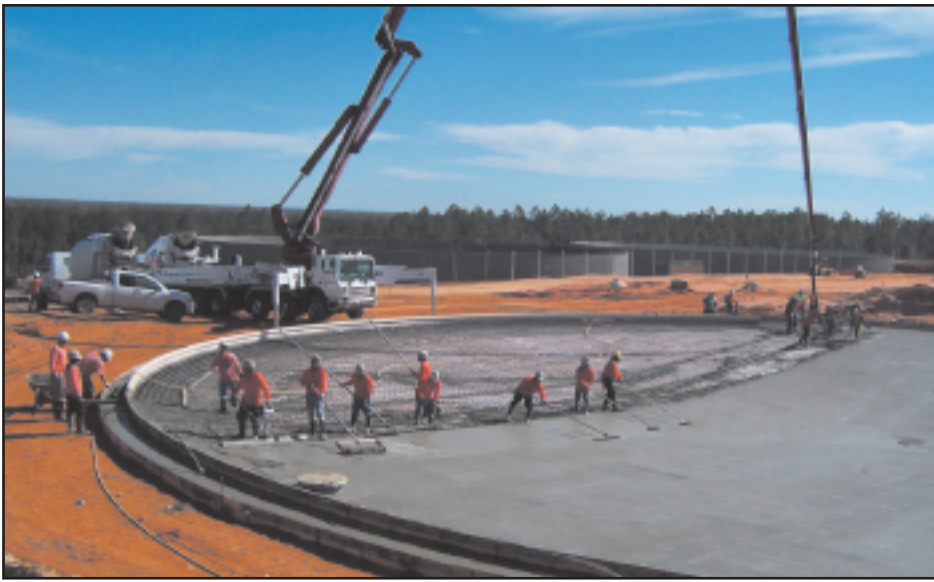
Construction of the prestressed concrete tank at the Central Water Reclamation Facility in February.
